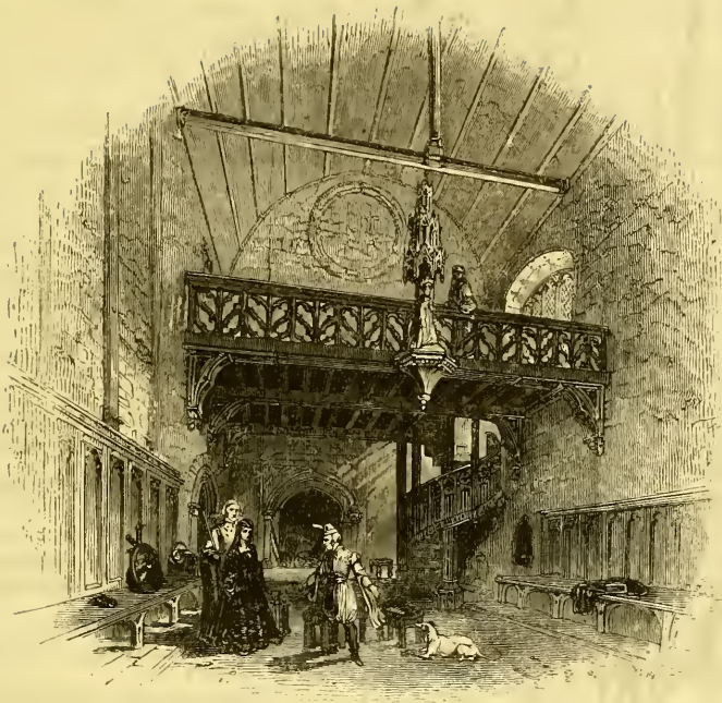
• [Interior of Palace in Rousillon.]
